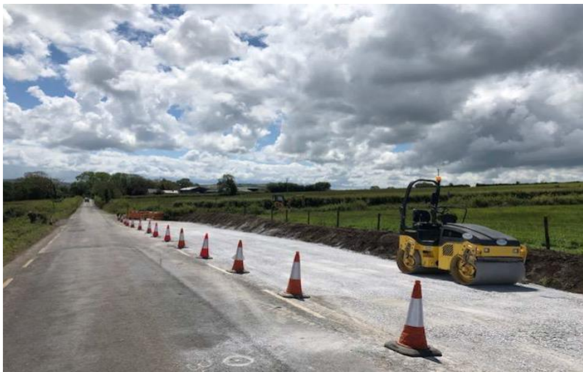
Plate 5.7 Passing Bay in Construction
