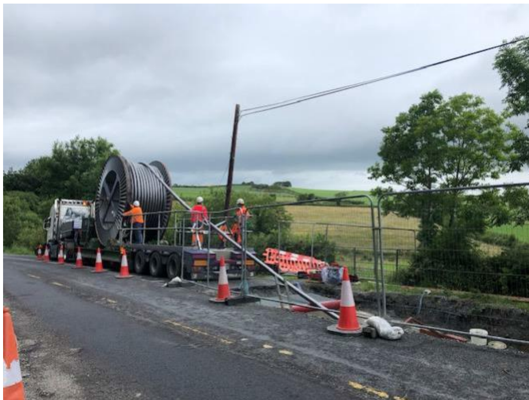
Plate 5.11 Typical Cable Pulling at a Joint Bay
