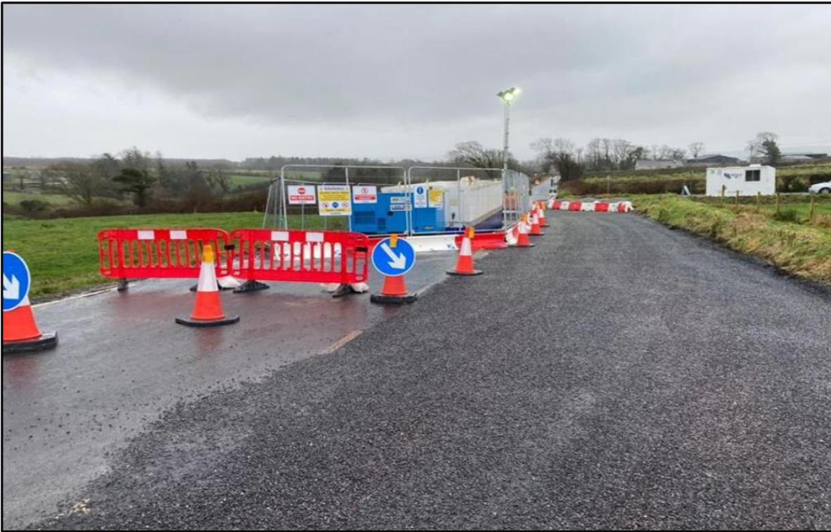
Plate 5.4 Typical passing bay – ensuring road traffic continues around a working area and joint bay
