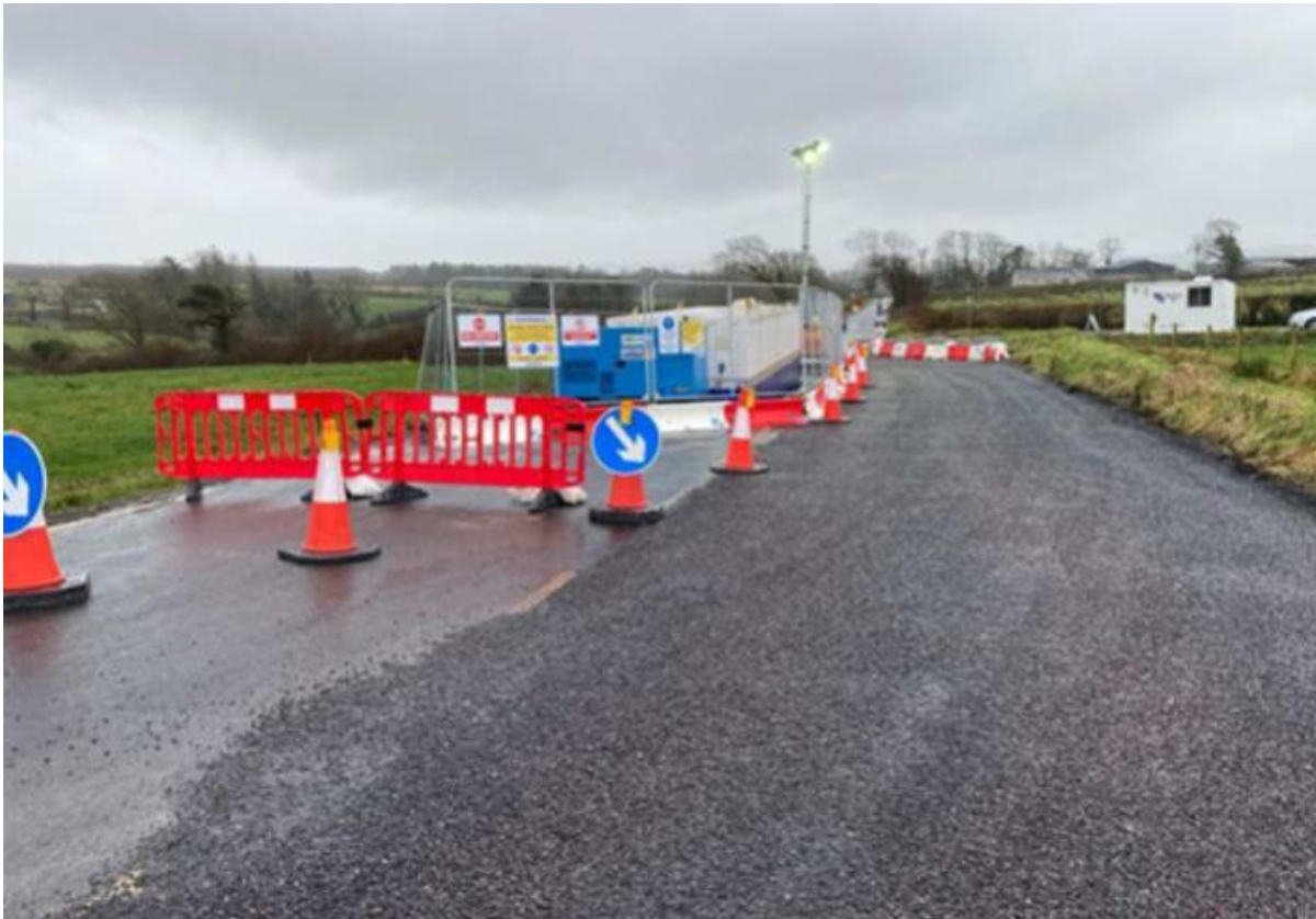
Plate 5.8 Operational Joint Bay with Passing Bay
