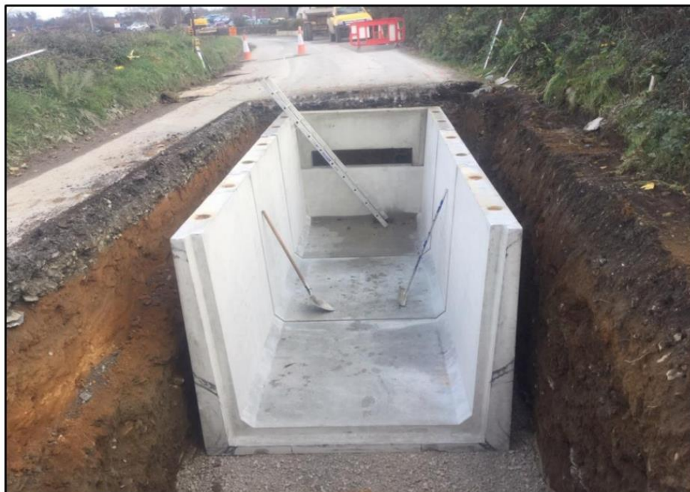
Plate 5.2 Typical Joint Bay During Construction
