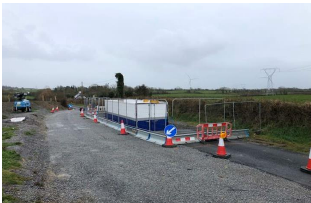
Plate 5.12 Typical Cable Jointing Bay Shelter
