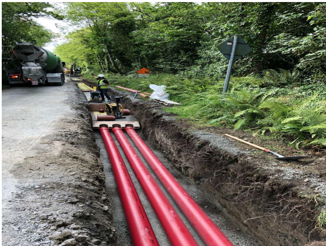
Plate 5.5 Proposed Cable Trench In-Road
