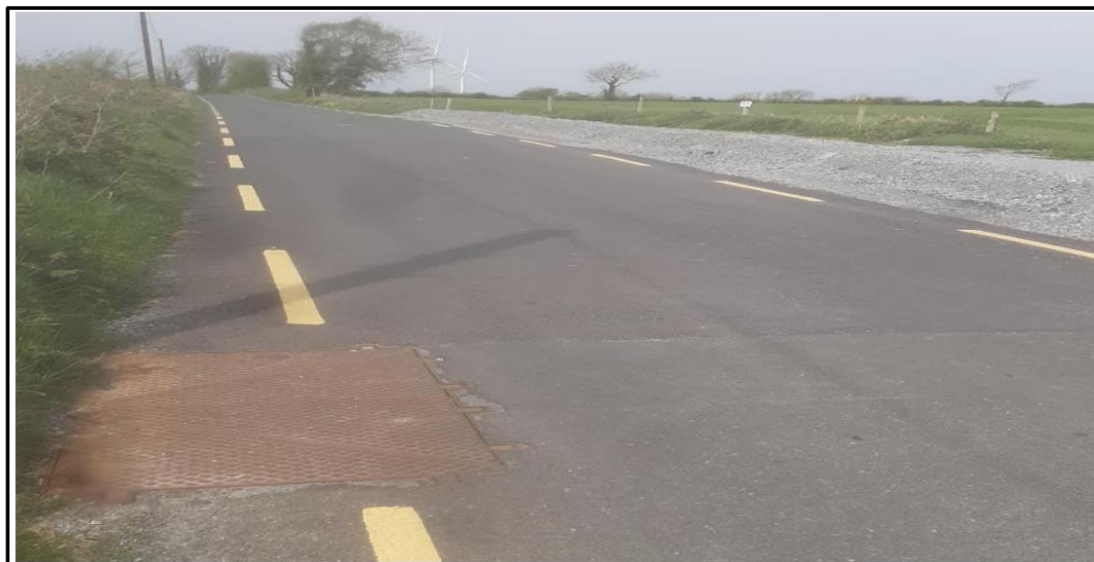
Plate 5.3 Reinstated road over joint bay (darker tarmac) with C2 communications chamber (steel chamber cover)
