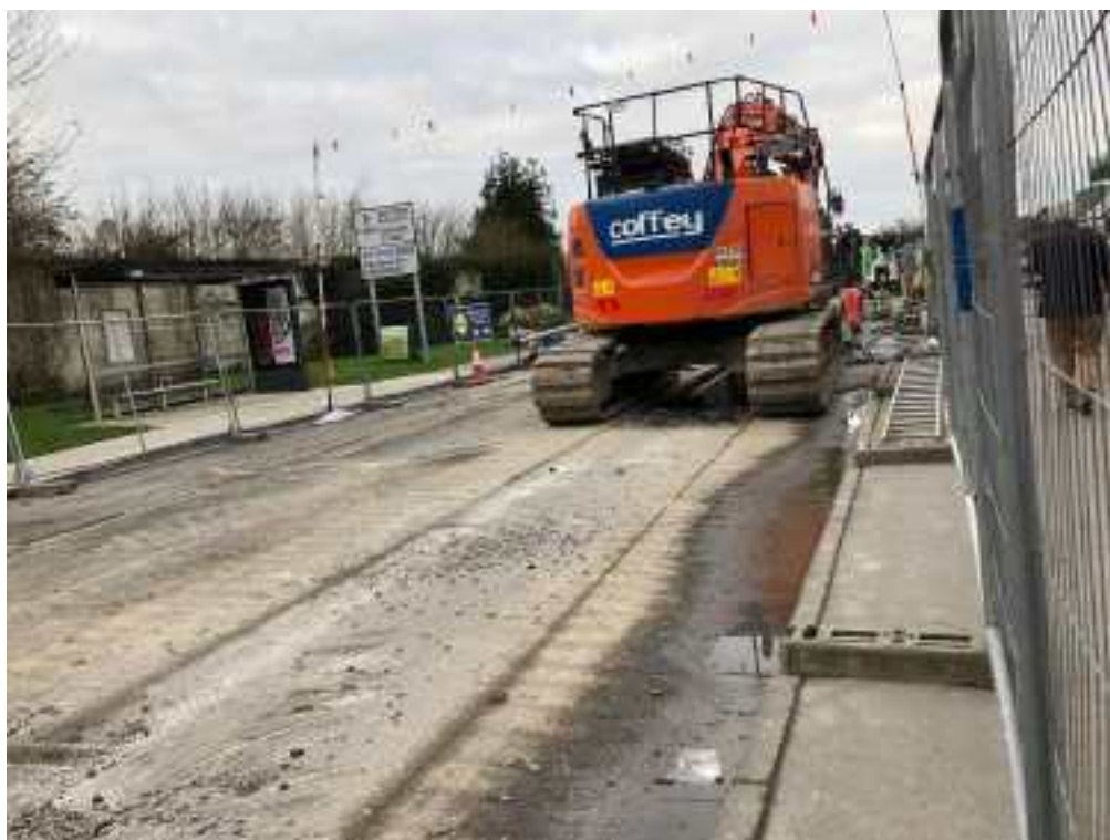
Figure 5-2 Preparation for removal of wearing course
