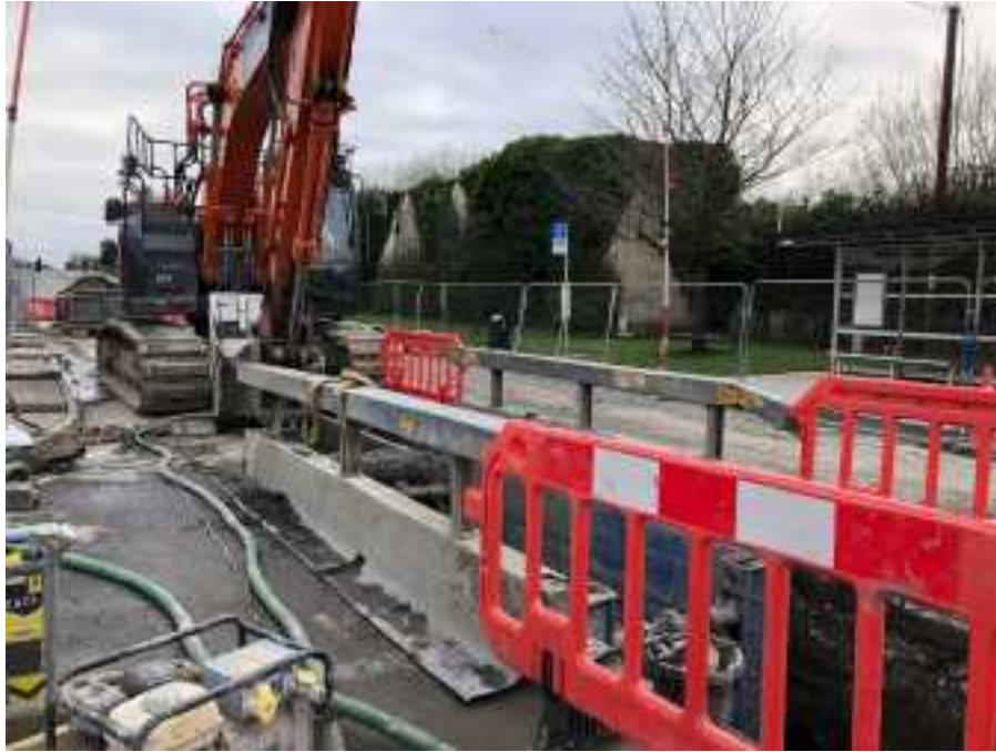
Figure 5-3 Excavation with trench box support
