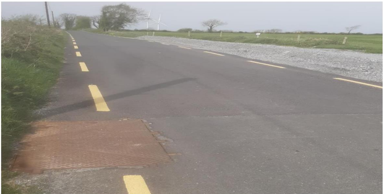
Image 2: Example of a proposed reinstated road over a Joint Bay (darker tarmac) with the C2 chamber cover visible
