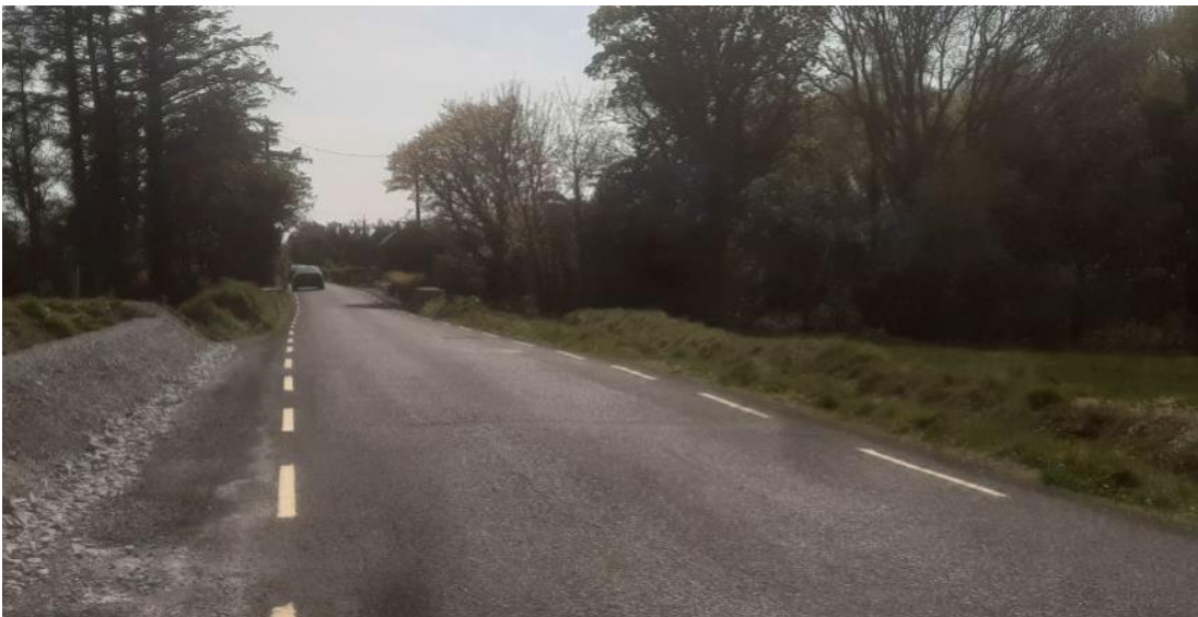
Image 5: Example of a Reinstated Road Following the Laying of Underground Cables
