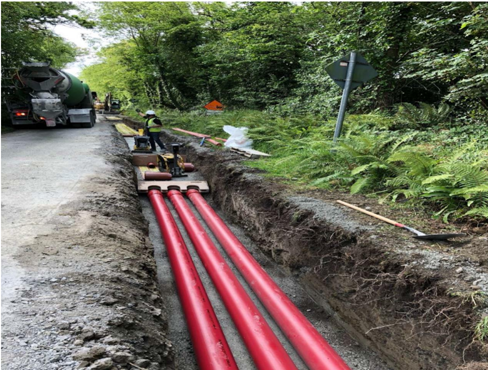
Image 4: Example of a Proposed Cable Trench In-Road with Cables in Flat Formation.
