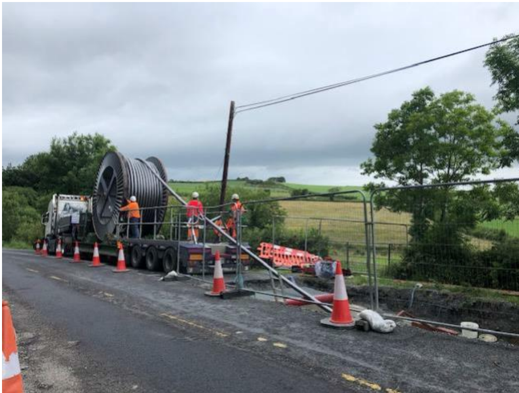
Plate 5.14: Typical Cable Pulling at a Joint Bay
