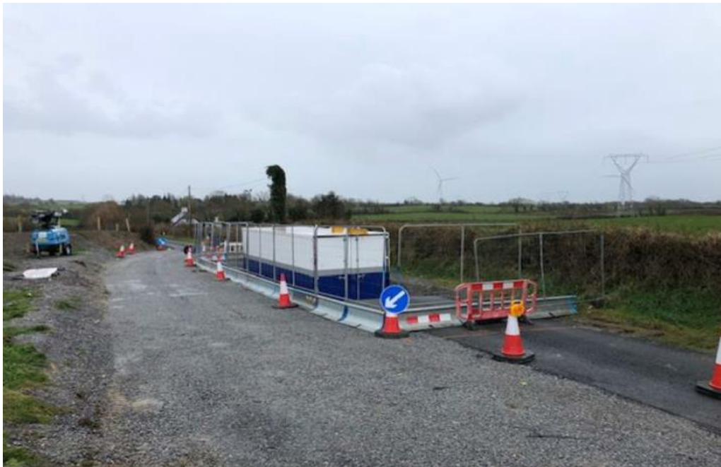
Plate 5.15: Typical Cable Jointing Bay Shelter
