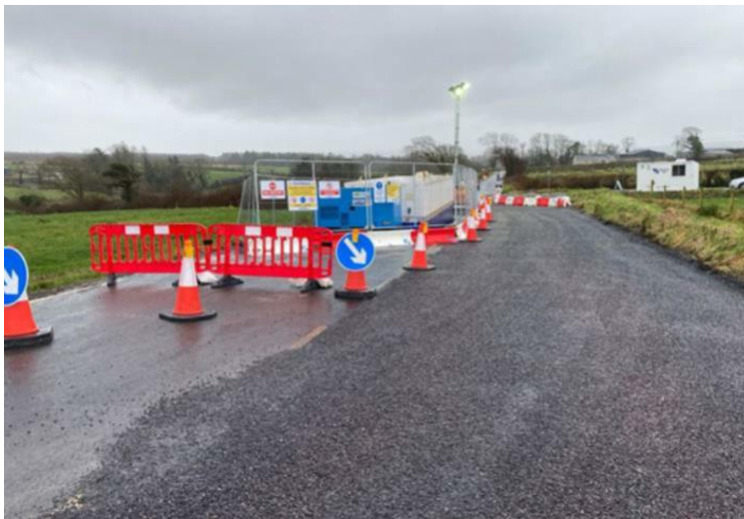
Plate 5.10: Operational Joint Bay with Passing Bay
