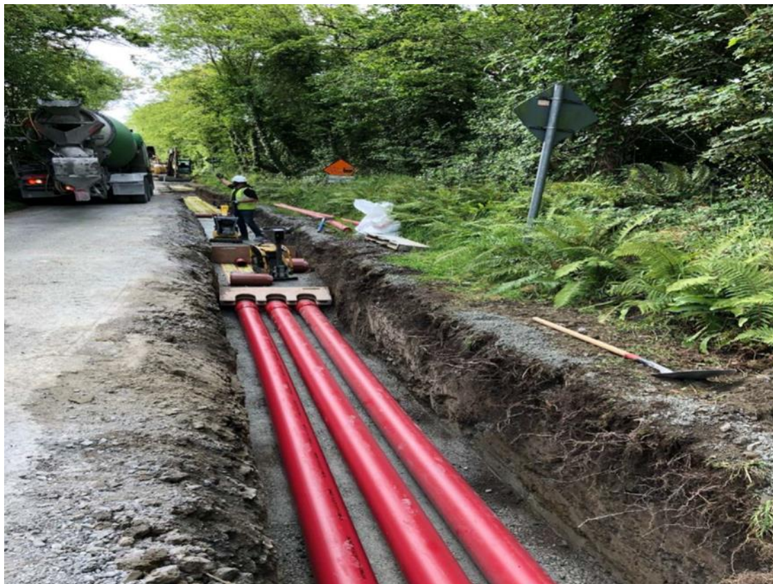
Plate 5.7: Proposed Cable Trench In-Road
