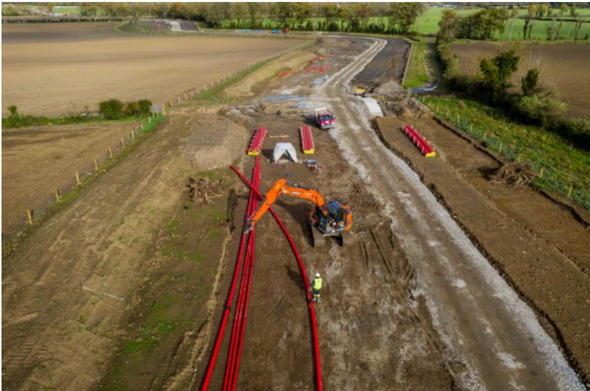
Plate 5.12: Typical Underground Cable Construction in Agricultural Lands
