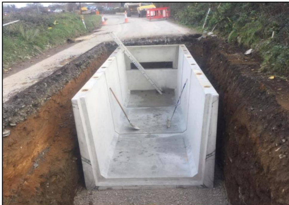
Plate 5.2: Typical Joint Bay During Construction
