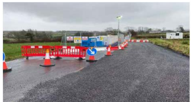
A typical passing bay in operation during cable jointing
