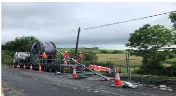
Cables being pulled into the ducts and jointing bay
