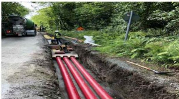
A typical cable duct installation in the road
