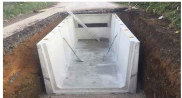
A typical jointing bay where cables are connected
