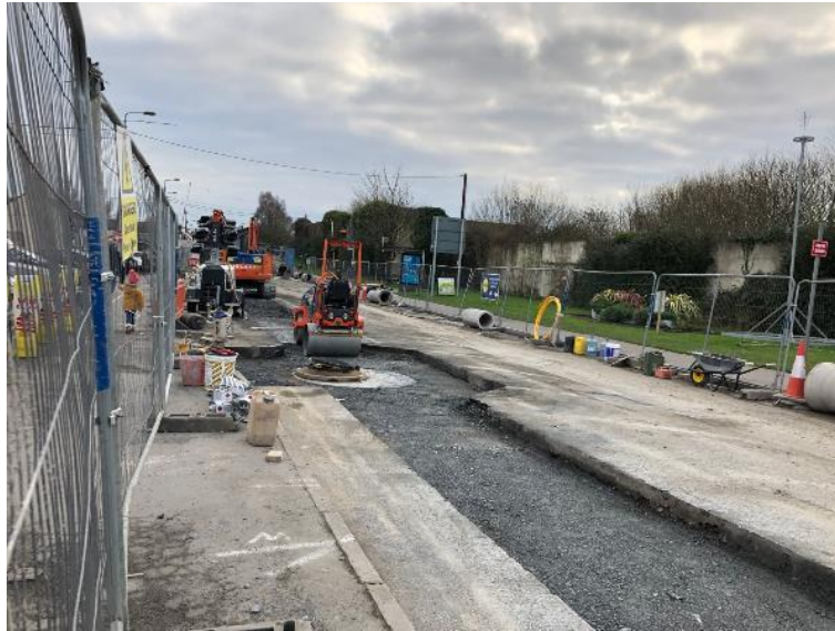
Figure 5-6 Resurfacing and backfill
