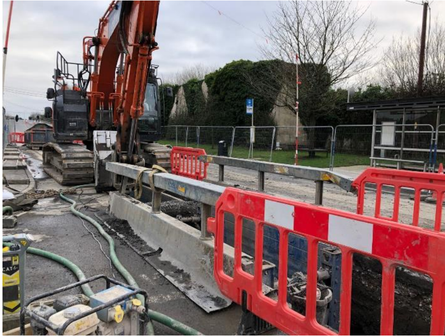
Figure 5-3 Excavation with trench box support
