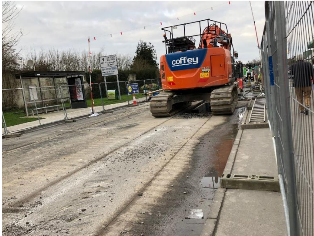
Figure 5-2 Preparation for removal of wearing course
