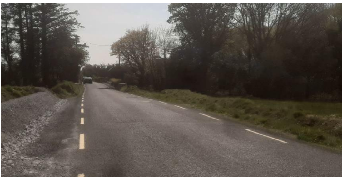
Image 5: Example of a Proposed Reinstated Road Following the Laying of Underground Cables
