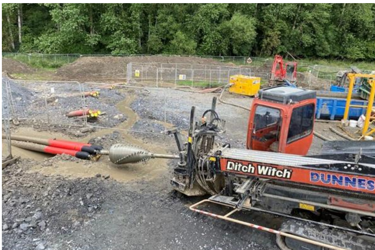
Image 6: HDD Receiving Pit with 220kV Cable being pulling through trenchless duct (Source LinkedIn – Pat Dunne, Dunnes Drilling Services Ltd).
