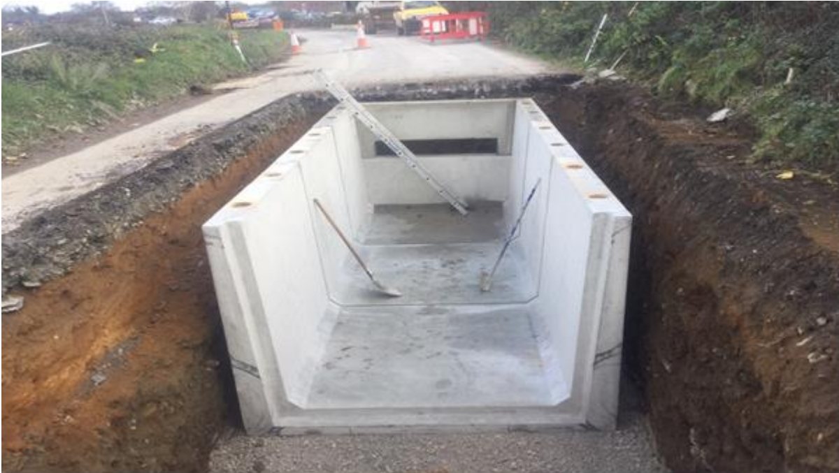
Image 1: Proposed Arrangement for a Joint Bay in Public Roadway.
